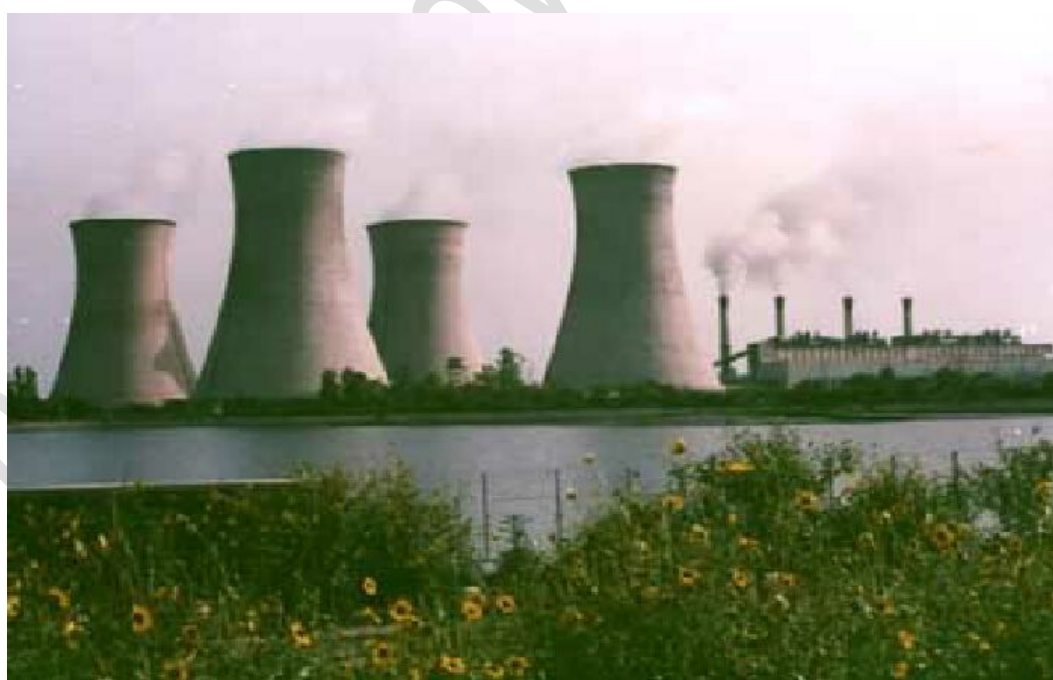
Figure 3: Thermal Plant, Bathinda
