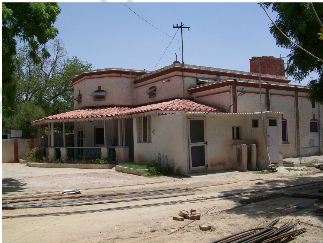
Figure 28: Residence of XEN Irrigation, Bathinda
